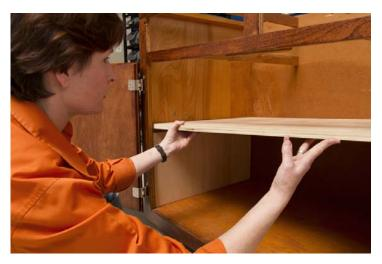
**2.** If you have a half shelf in the back of the cabinet, you can keep it and install the pullouts only on the bottom, or you can cut the shelf in half to make it easier to remove.
