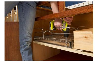
To install, set your pullouts in the cabinet space and verify that they will not bump into framing or hinges when you pull them out. When you're satisfied that they will function properly, mark the mounting holes (typically two front and two back) with a pencil on the shelf. You can then remove the shelf from the mounting assembly if needed to install the screws. Once all mounting screws are in place, reinstall the pullout shelf and test it out.
