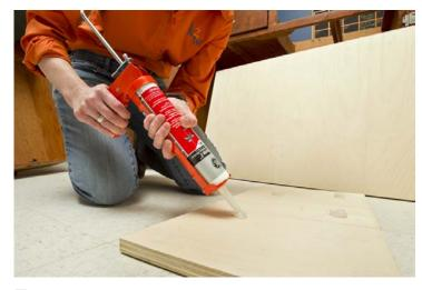
**3.** You can use a silicone adhesive to hold the shelf supports in place on both ends. Just apply several large (1-inch) dots of silicone on the surface and press firmly into place. This will spread the silicone and hold it in place as the adhesive dries. Set the shelf directly on top of the shelf supports. Hardware is not required, but if you choose to use nails or screws, make sure you will not pierce the exterior of the cabinet with nails that are too long.
