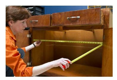
**1.** Measure the opening in your cabinet, left to right. For cabinets with a face frame, the opening is between the face frame, not the available space behind the frame. For cabinets with no face frame, it is the actual interior space. For both, minus space for any hinges that may be bumped by the pullouts.
